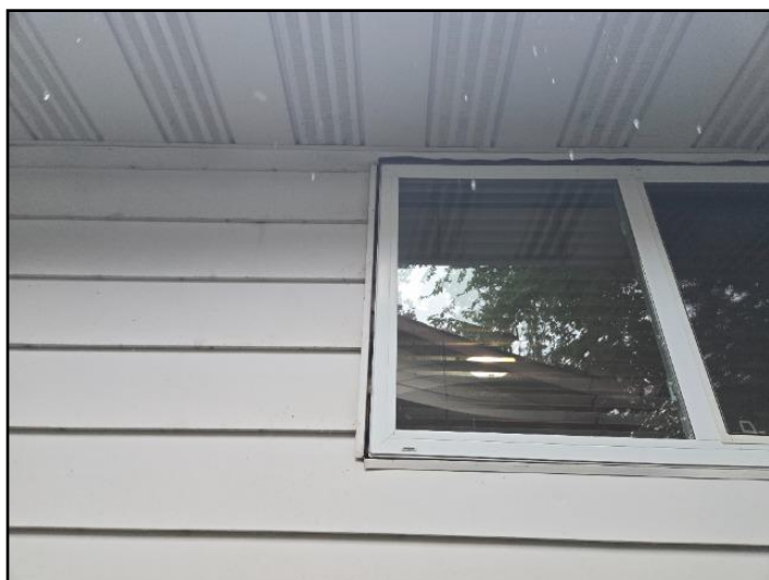
Sealant missing
