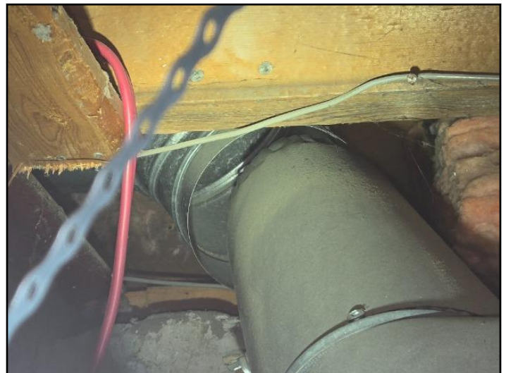
Disconnected ducts
