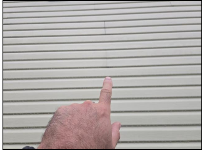
Joint separation
