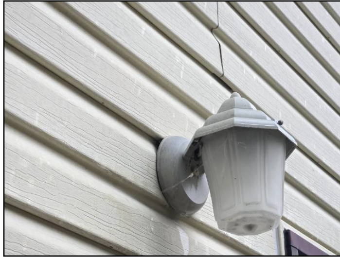
Sealant missing
