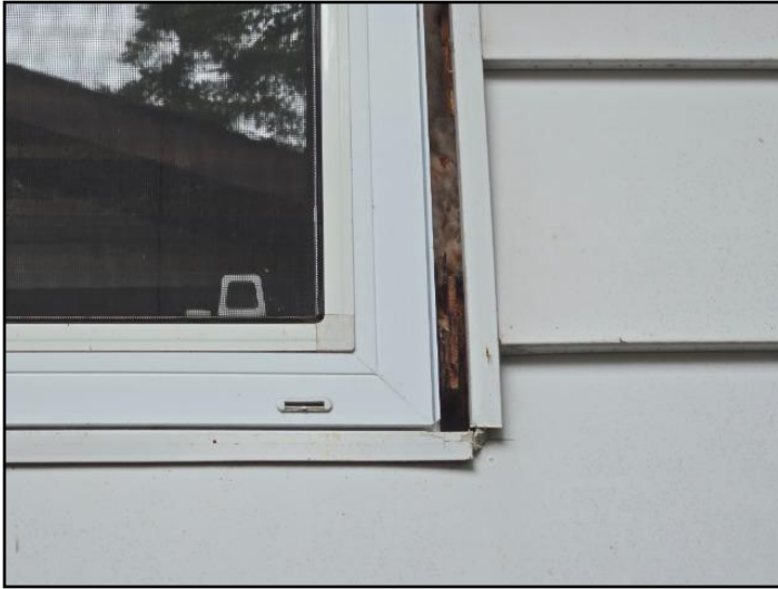
Sealant missing
