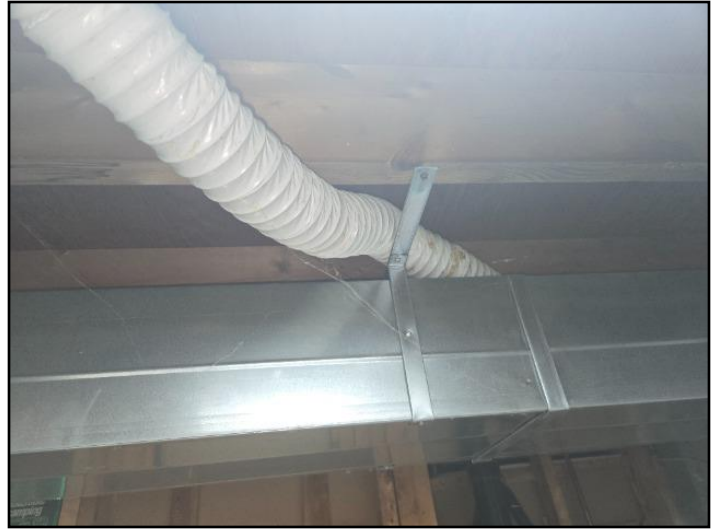
Poor connection
