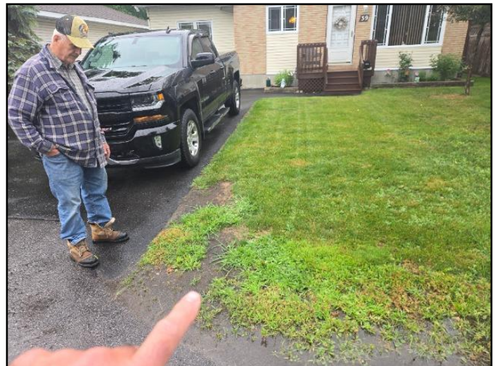
Discharge pipe problems
