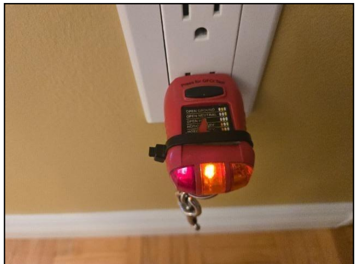
Reversed polarity Front door
