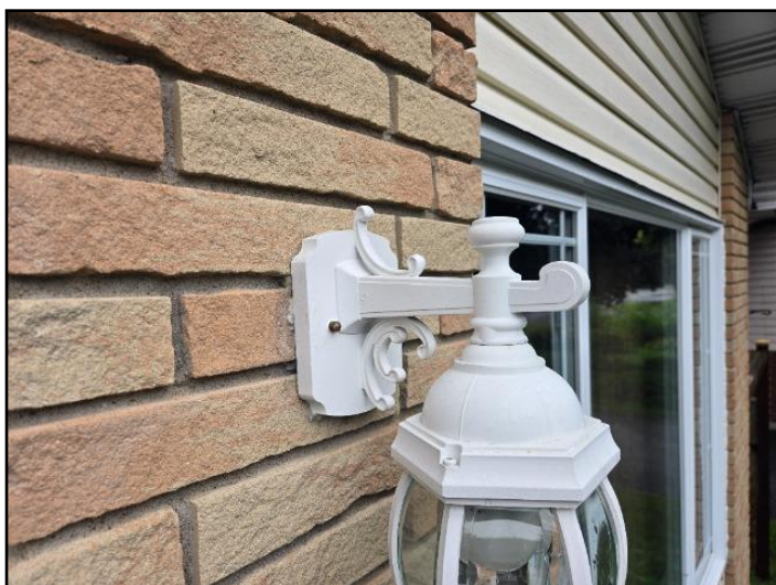
Sealant missing
