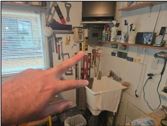
Box location poor
