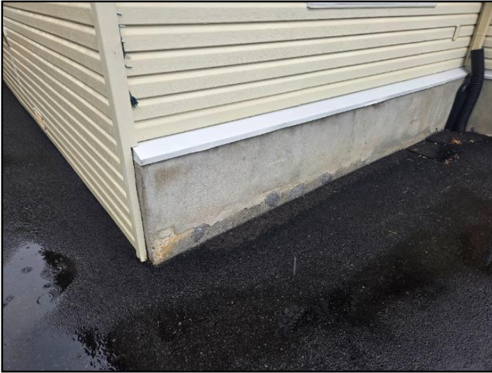
Parging damaged
