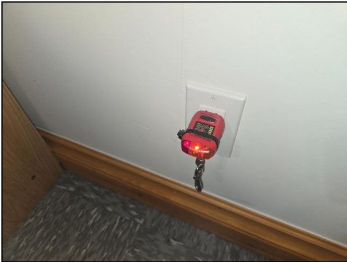
Reversed polarity Basement
