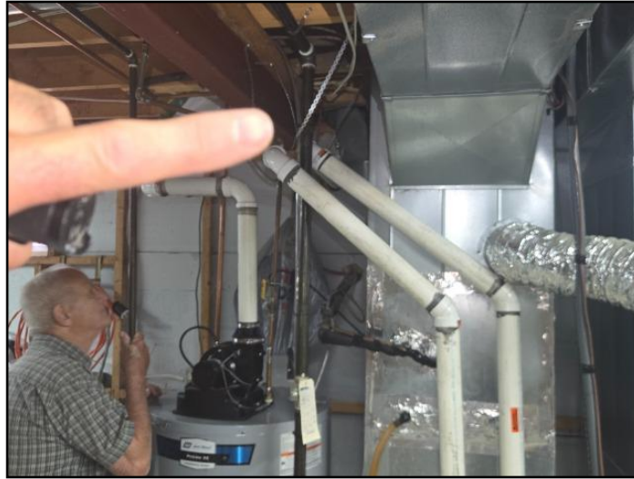
Disconnected ducts
