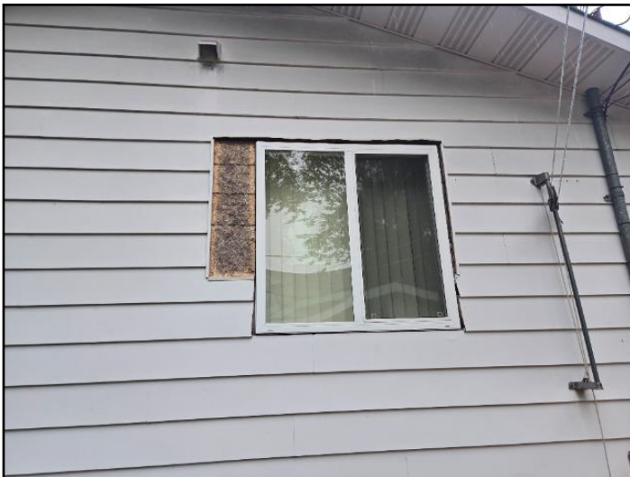
Sealant missing
