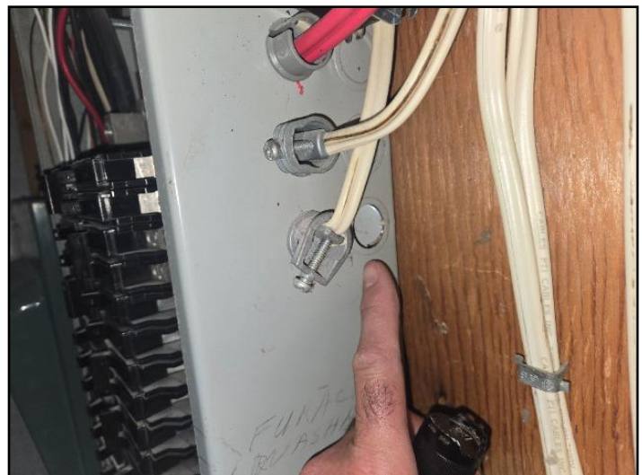
Unprotected openings
