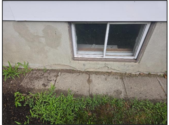
Parging damaged
