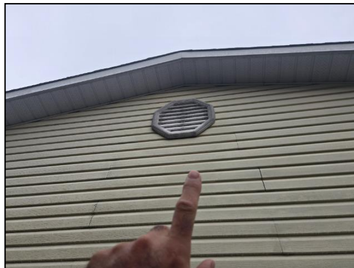
Joint separation
