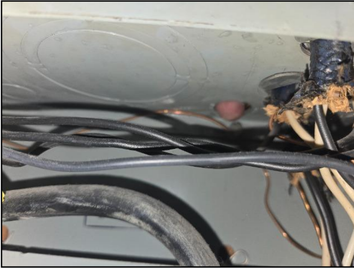
Unprotected openings
