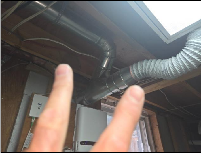
Poor connection
