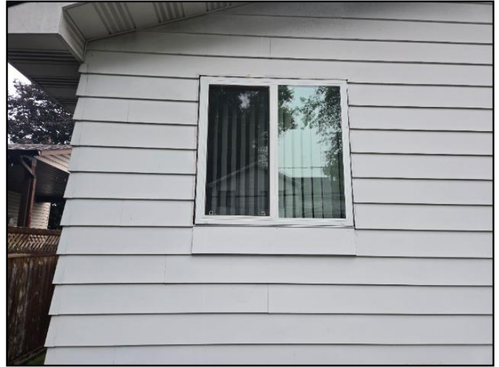
Sealant missing
