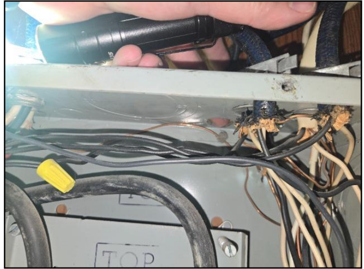
Unprotected openings
