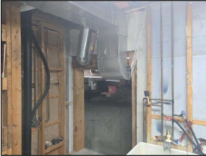
Entrance to crawl space
