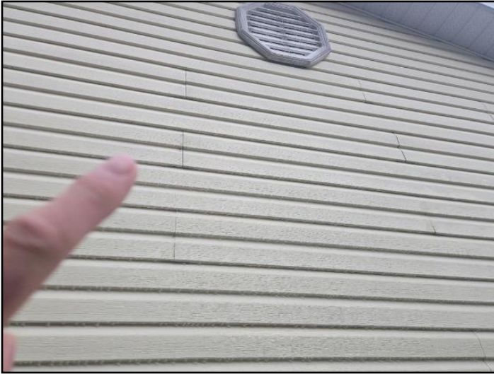
Joint separation
