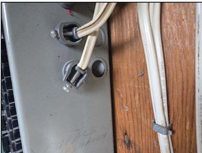
Unprotected openings
