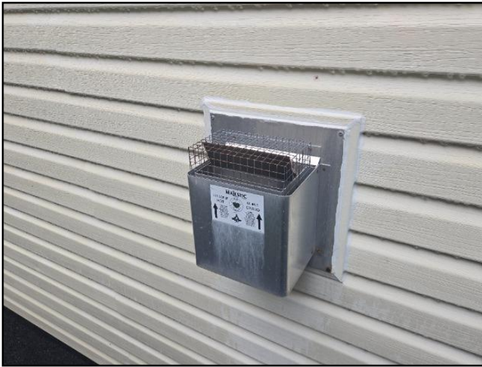
Direct vent clearance
