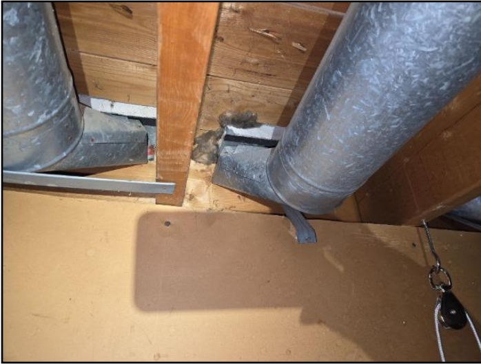
Disconnected ducts
