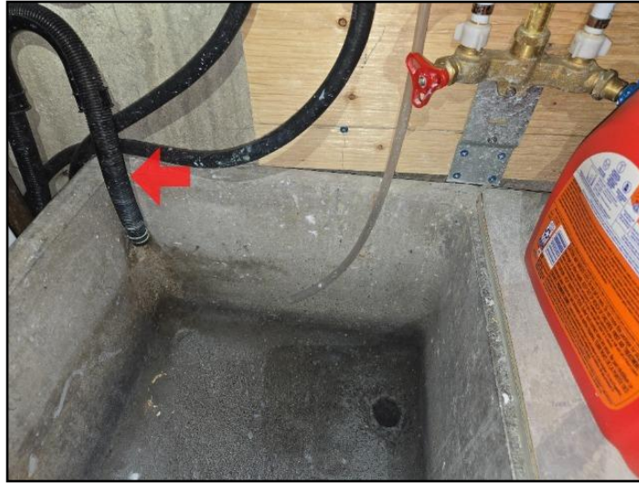
Standpipe missing
