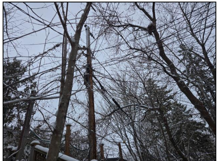
Branches / vines interfering with wires
