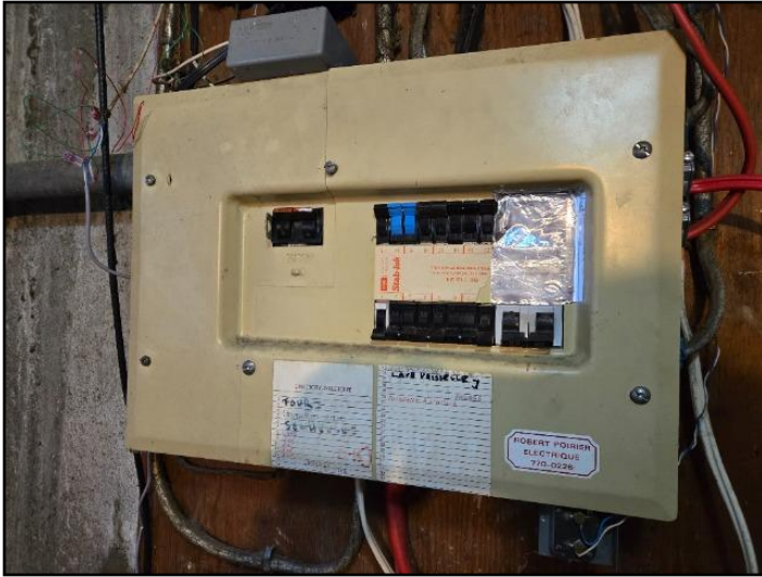
Aging Federal Pioneer/Stab-Lock
