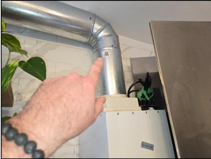
Poor connection
