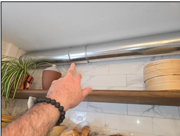
Poor connection
