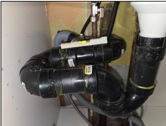
Insufficient slope
