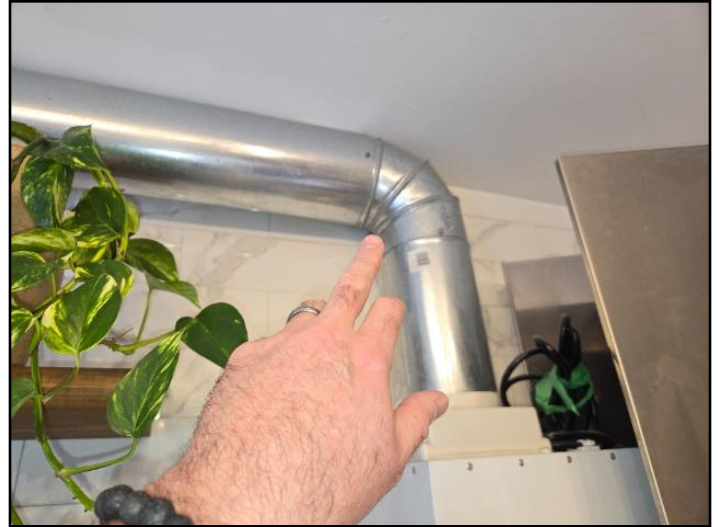
Poor connection
