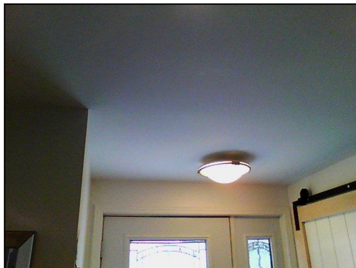
Gaps or voids
