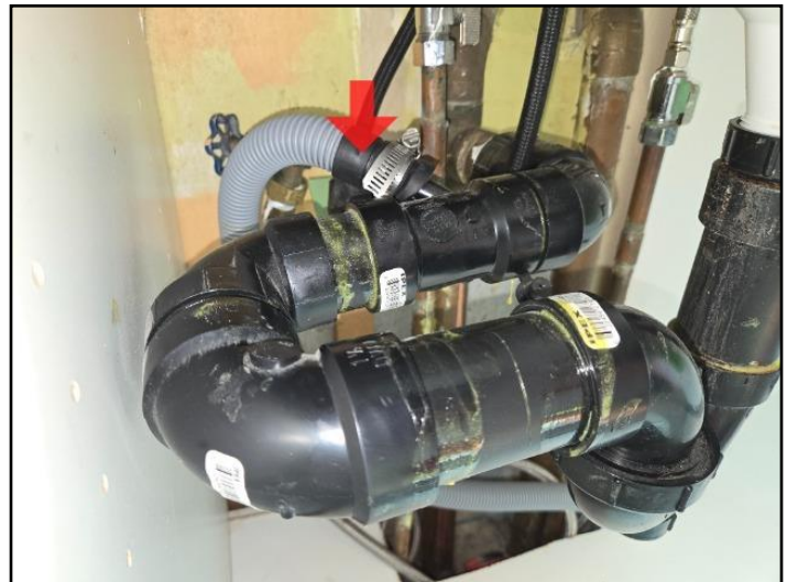
Dishwasher drain connections
