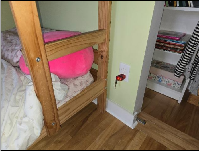
Reversed polarity
