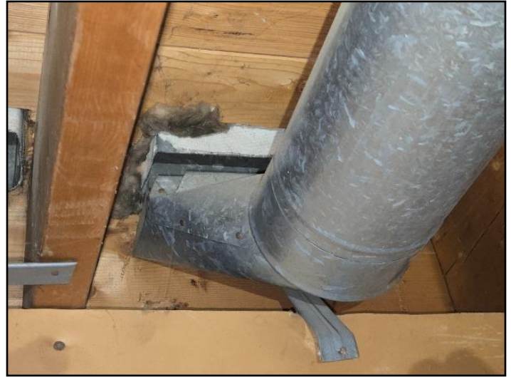
Disconnected ducts
