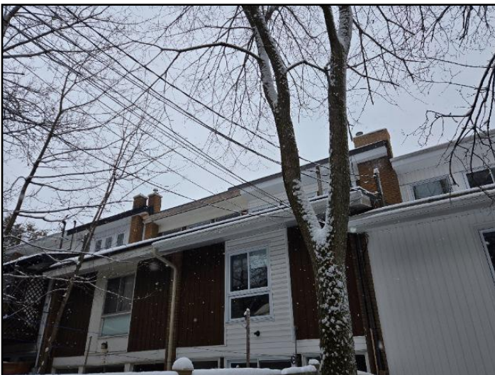
Branches / vines interfering with wires
